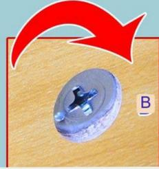
Turn the eccentric bolt clockwise to lock the board
