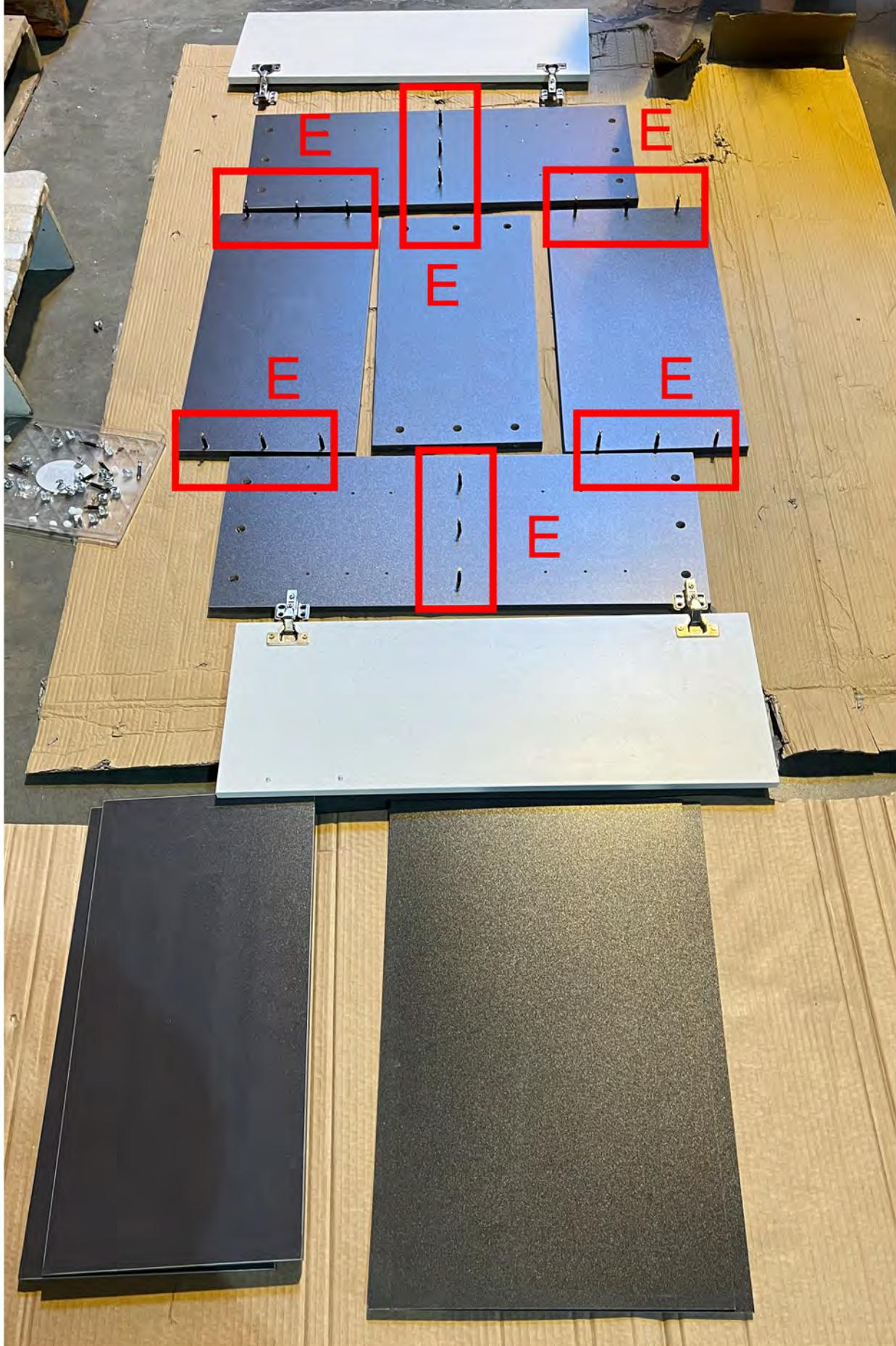
Tighten E into all white pre-installed inserts. Do not overtighten—stop once resistance is felt and the fitting is secure without looseness. Ensure vertical installation as much as possible.
