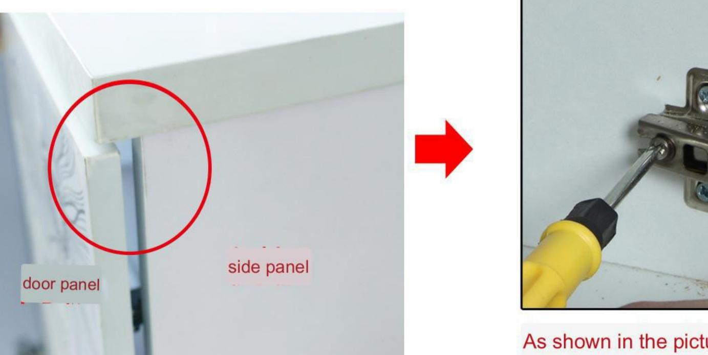
As shown in the picture, loosen the screw pointed by the screwdriver, push the door panel in or pull it out, and then
