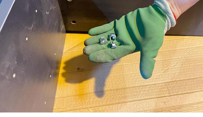
Secure part F into the large pre-drilled holes. Refer to the "Instructions for Using Eccentric Bolts" for detailed guidance.
